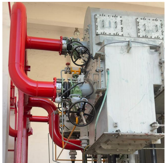
Comprehensive transformer modification and safety upgrades executed by Anpec
