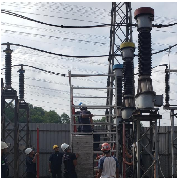
Anpec engineering personnel executing substation construction and installation works
